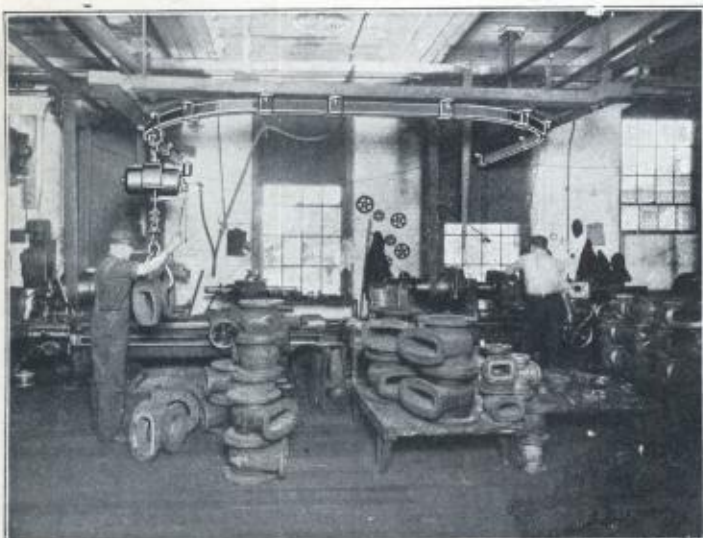
Over-Way facilitates handling heavy castings
